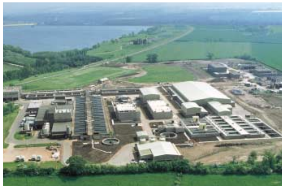
Figure 5: Anglian Water's Grafham Water Treatment Works. Incorporating preozonation, final ozonation and Biflux GAC contactors.
